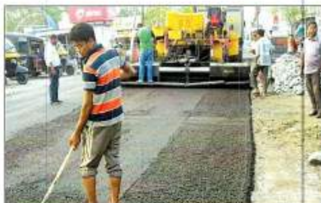
Laying of Cold Mix with Paver
