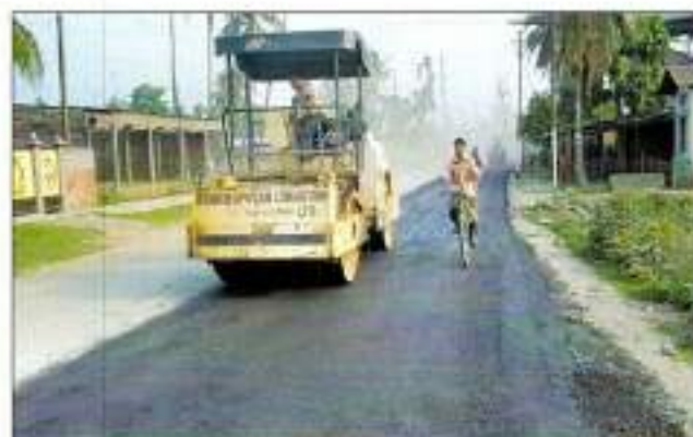
Compaction of Cold Mix
