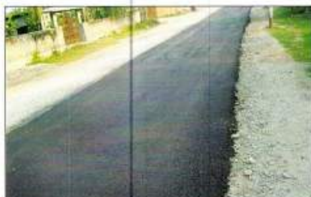
Cold Mix Road Finished Surface
